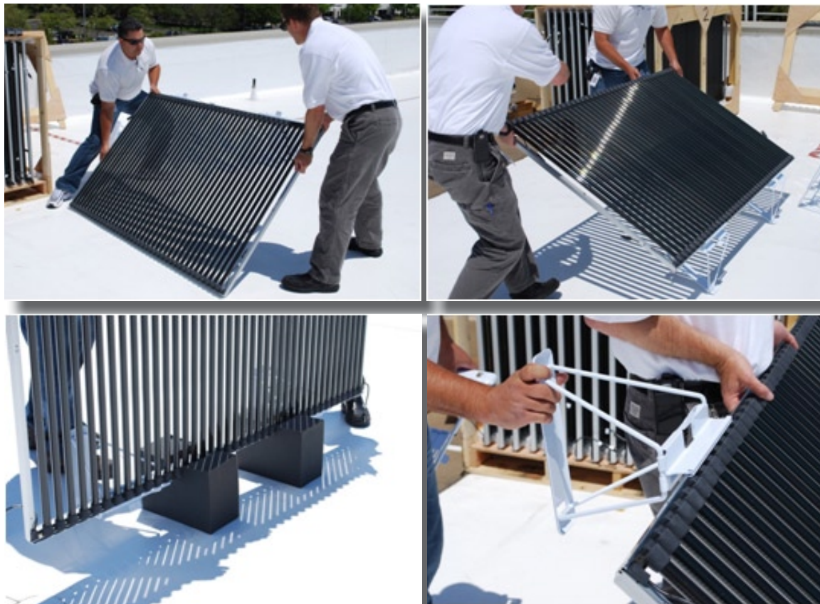
Figure 14. Adding Additional Mounts to First Panel
