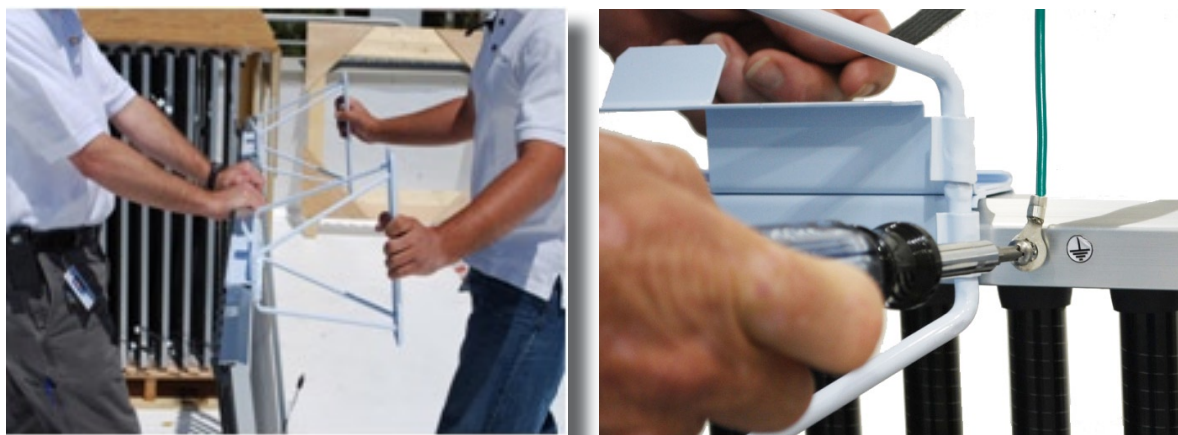
Figure 12. Attaching the First Two Mounts
