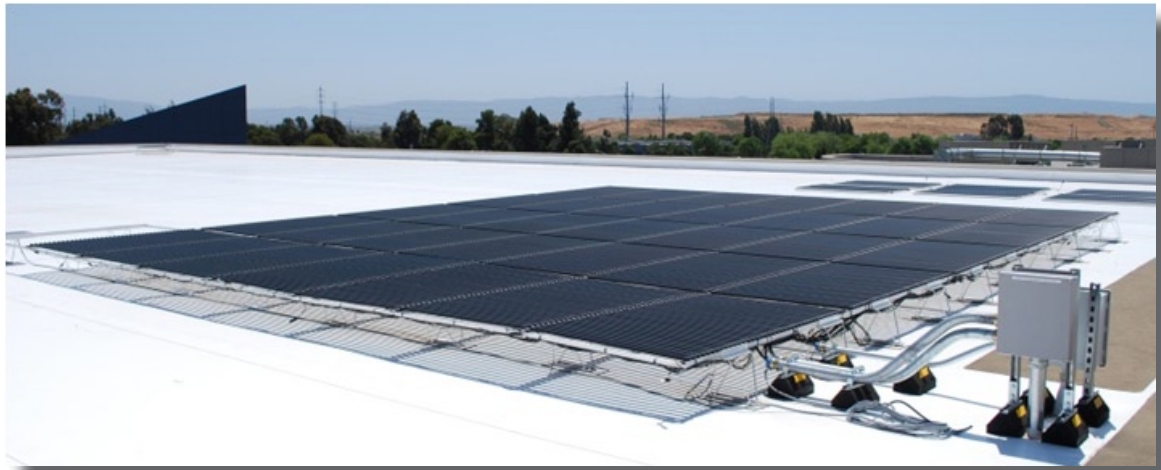
Figure 6. Typical Solyndra Photovoltaic Panel Installation
