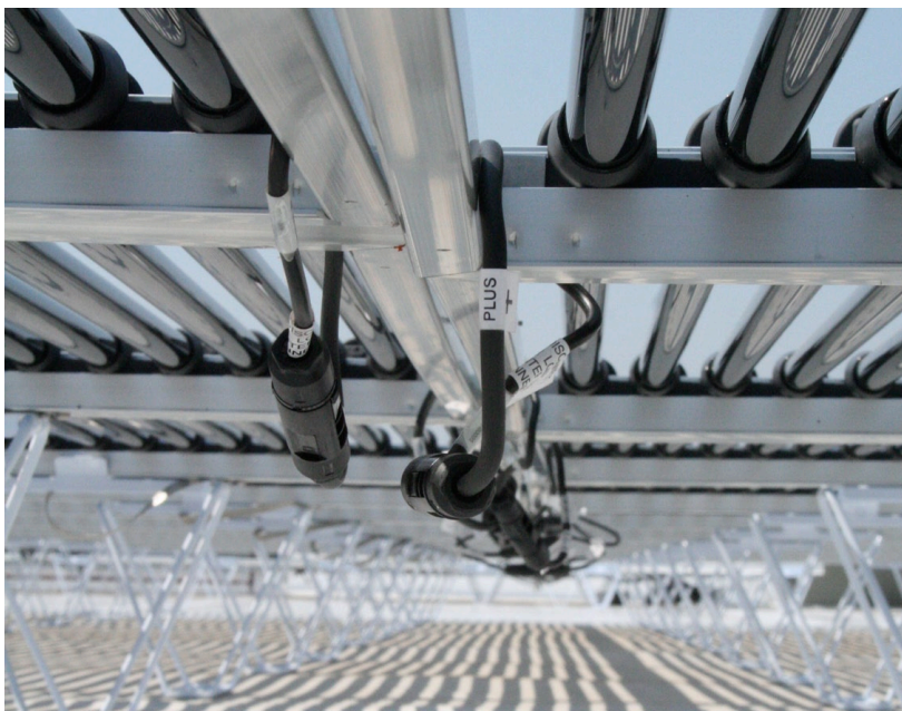
Figure 22. Interpanel Electrical Connections
