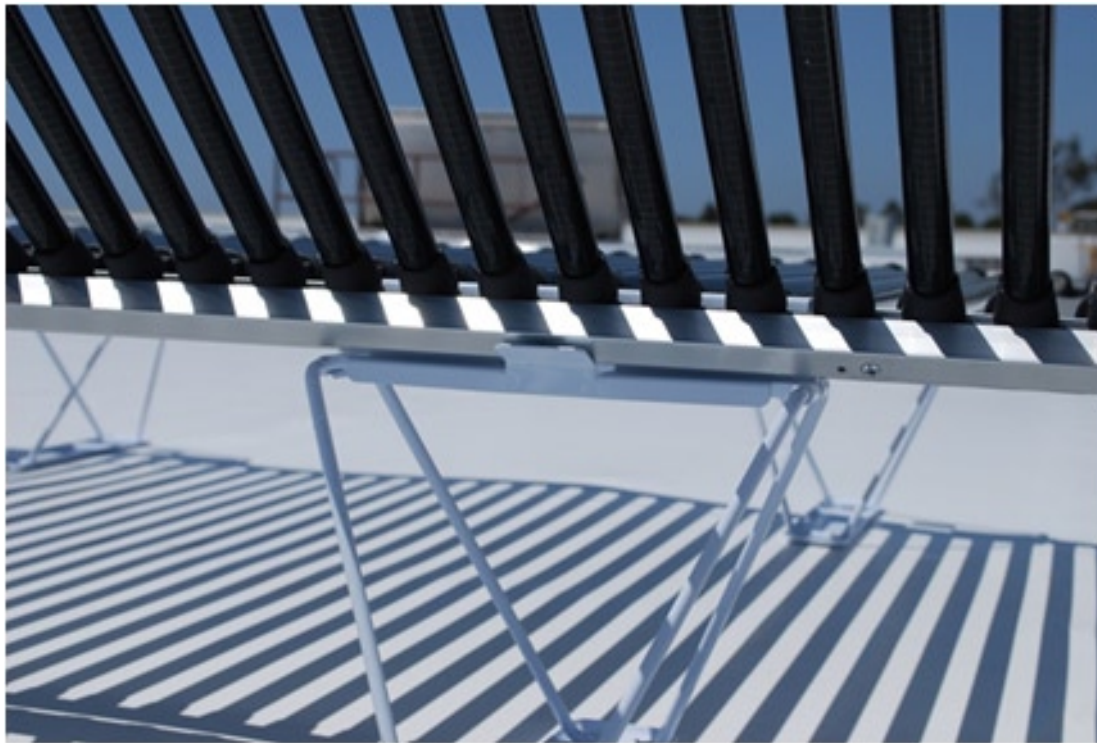
Figure 20. Joining the Panels - Angling Panel Up
