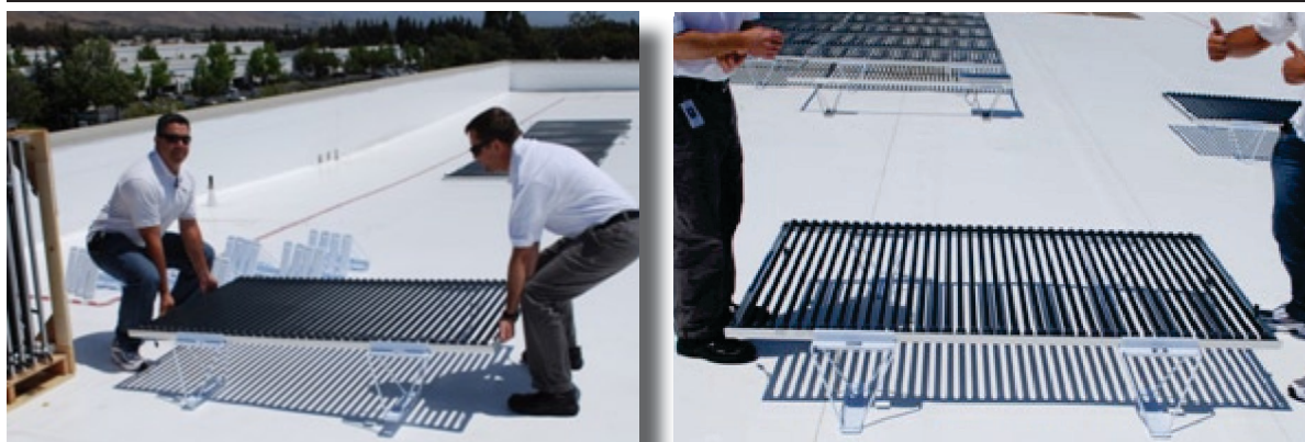
Figure 15. Placing the First Panel
