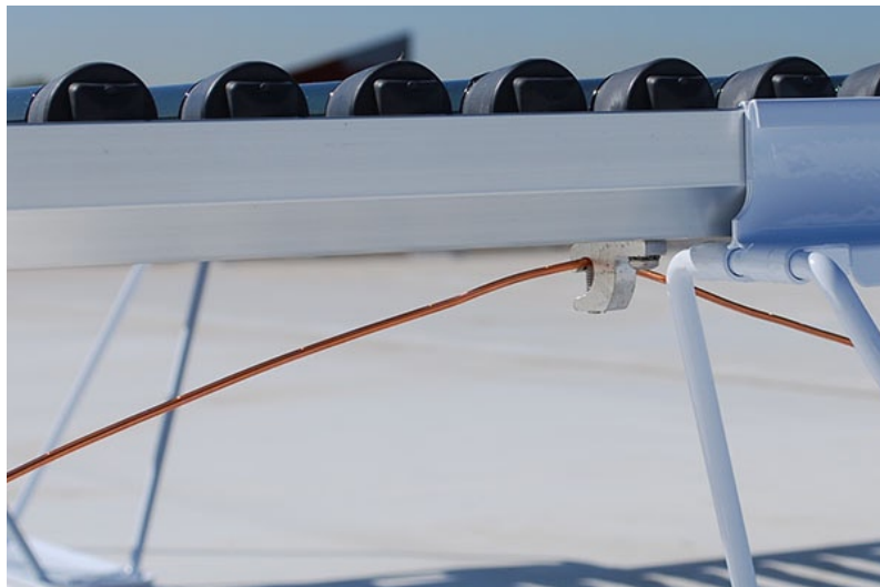
Figure 17. Installing the Ground Wire
