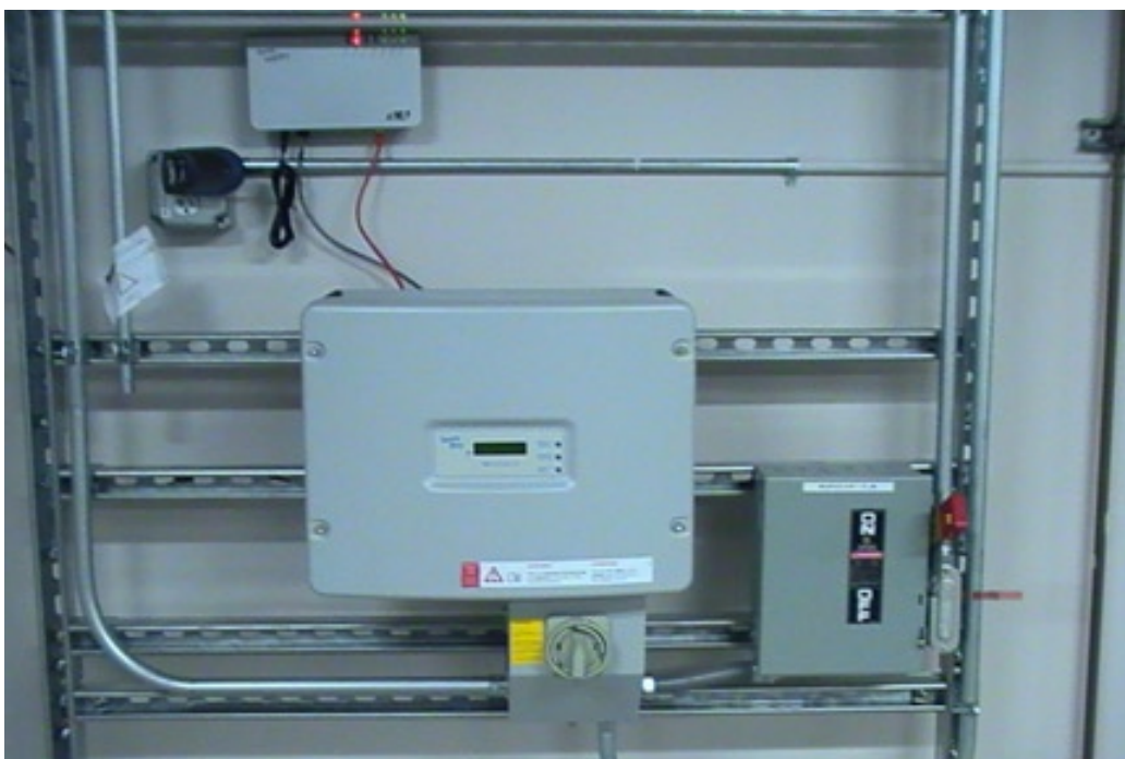
Figure 32. Typical Inverter Installation
