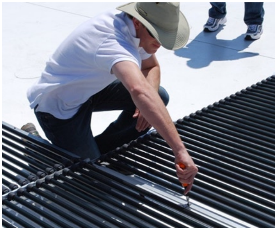
Figure 28. Lateral Clip After Installation
