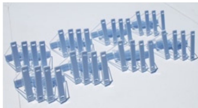
Figure 10. Panel Mounts, Staged for Installation
